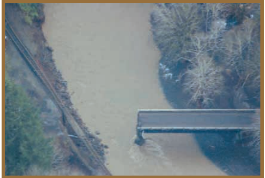
An aerial photograph from an Oregon Wing Cessna shows how floodwaters destroyed a bridge above the Lower Nehalem River. Damaged train tracks can be seen to the left of the broken bridge.
